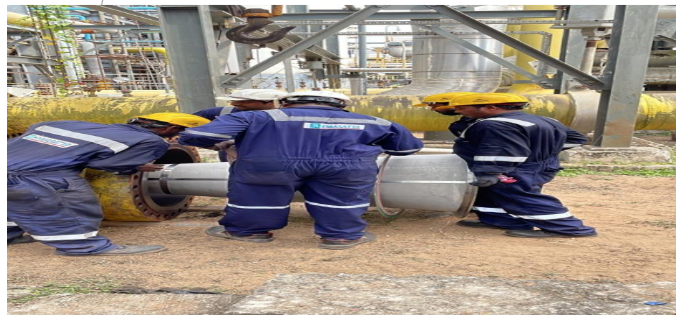
32" Strainer Erection at ONGC VA-S1, Odalarevu Onshore Terminal, Odalarevu
