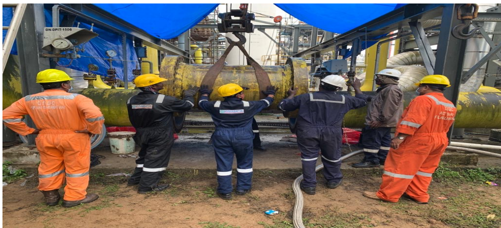
32" Strainer Erection at ONGC VA-S1, Odalarevu Onshore Terminal, Odalarevu
